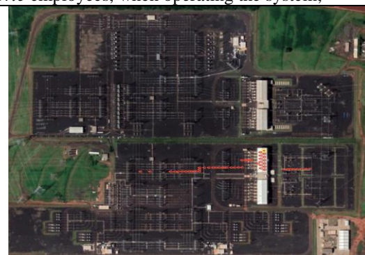
Figure 3- General View of HVDC Substation (ELN360)
