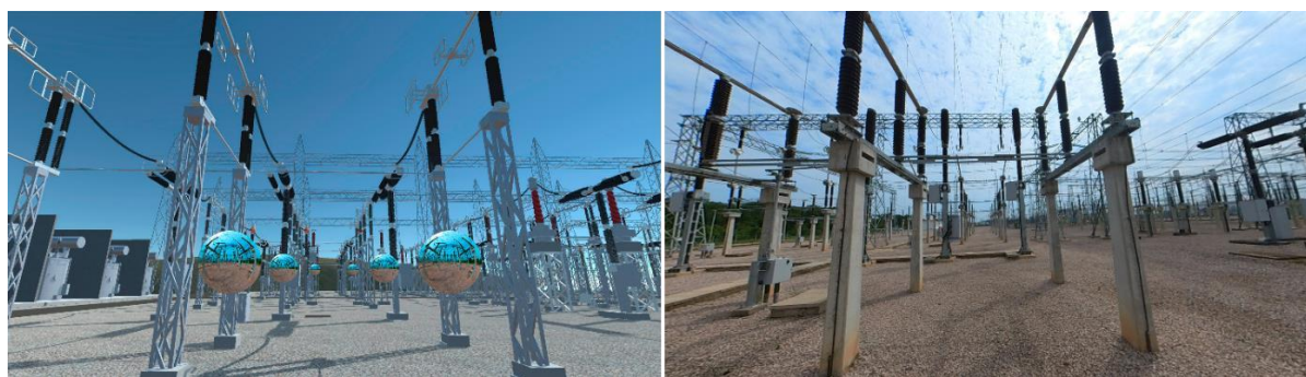
Figure 5- Virtual substation with inserted spheres (left) and a 360-degree photo opened in a specific position (right).
